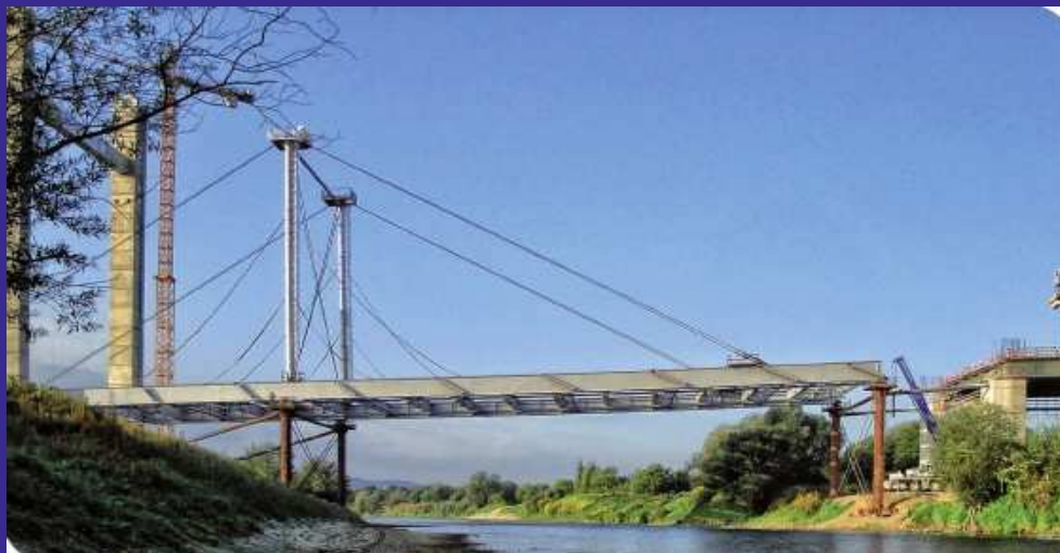
Construction of the suspended bridge over the river San in Przemyśl, provincial road connecting the National Road No. 77 and No. 28
