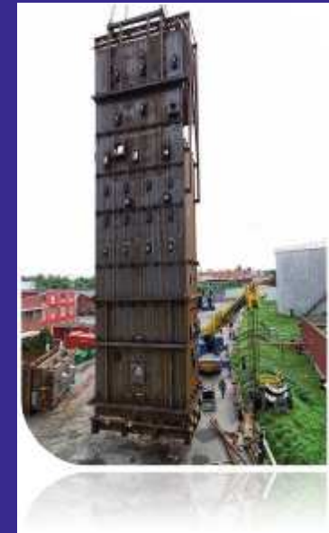
Installation of the boiler in E.On Värme Sverige, Örebro
