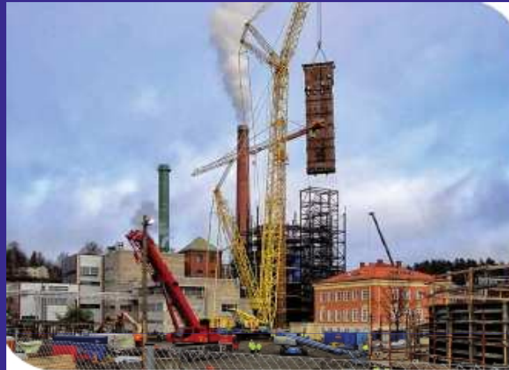
Installation of biomass boiler for power plant in Havo, Finland
