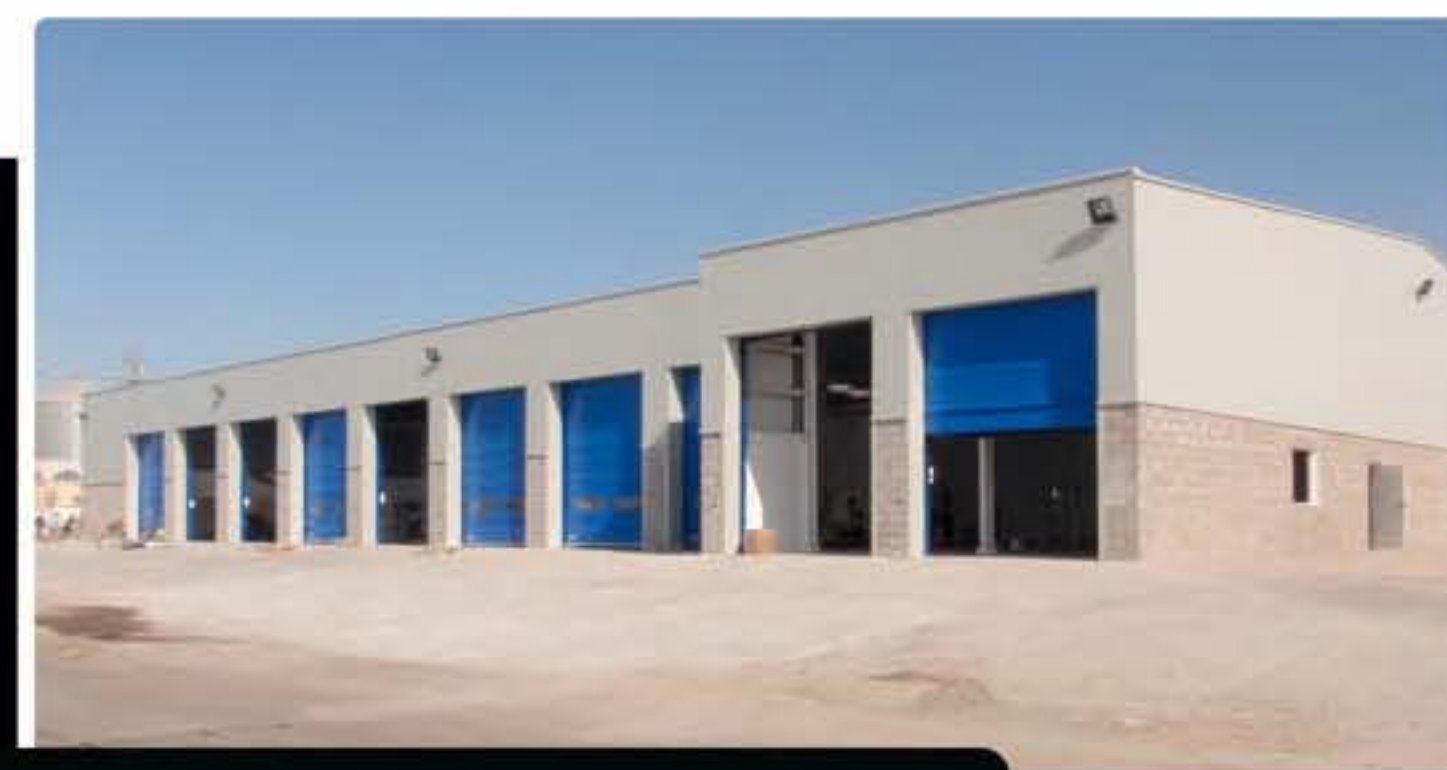
EMMSA | Nave taller para Alsa EMMSA | Workshop Bay Alsa
